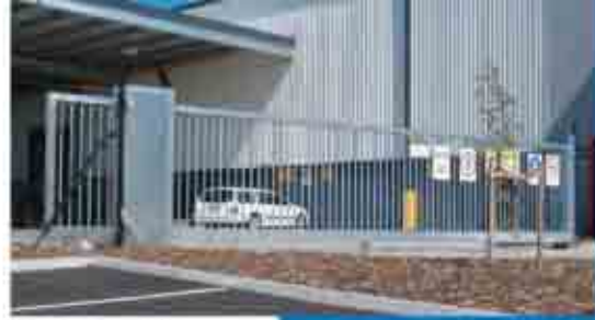
MTG - Slide gate incorporating ground tracks
