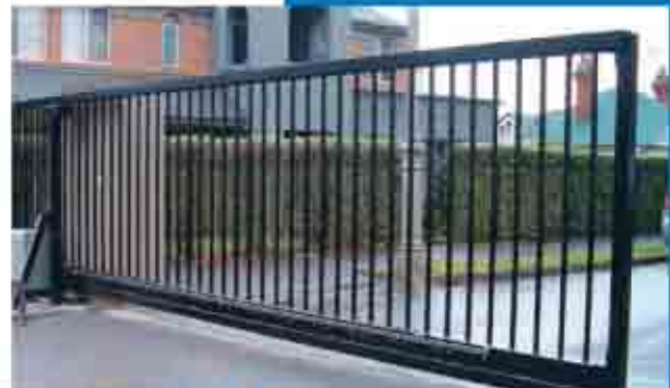
MSL - Cantilevered gates do not require either ground or above ground tracks
