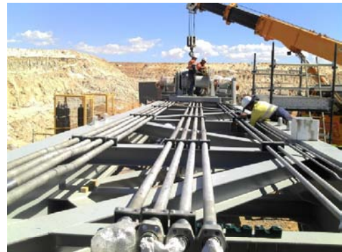
Tiwest Dredge Refurbishment
