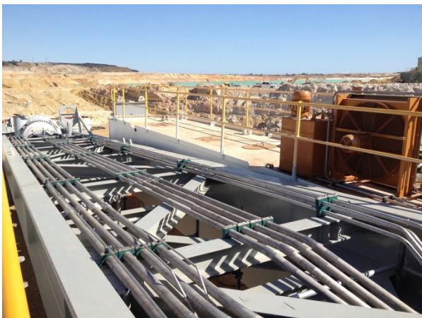
Tiwest Dredge Refurbishment
