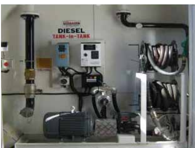
UPGRADES TO FMS & PUMPS
