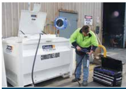
TANK & EQUIPMENT REPAIRS
