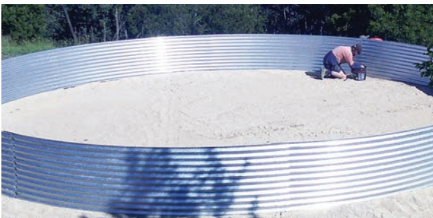
Construction at your site
