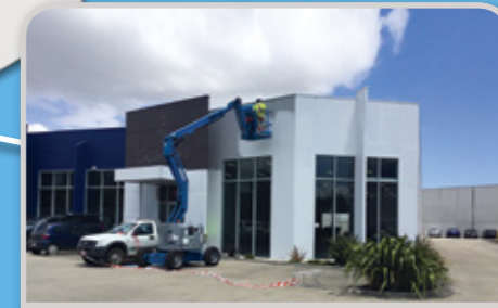
EXTERIOR FACADE REFACING & CLADDING
