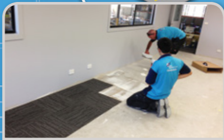
FLOORING (INC. CARPETS & TILING)
