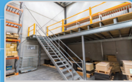
MODULAR RAISED STORAGE AREAS
