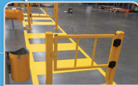
SAFETY BARRIERS & LINE MARKING
